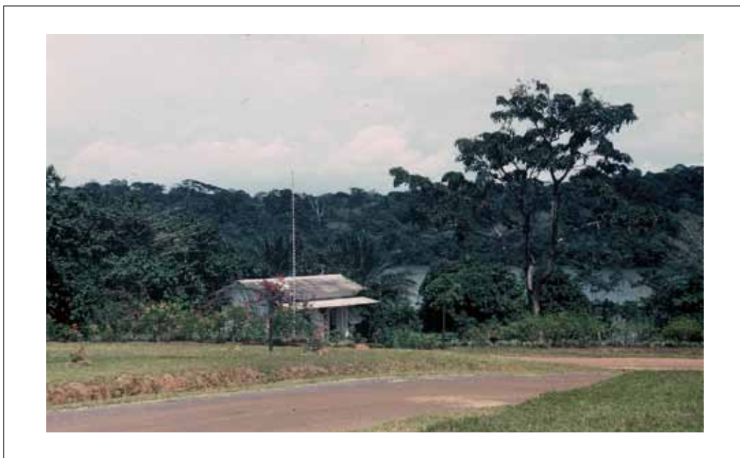
The CSRS's main building colloquially called "le clapier" [rabbit hutch], source: Hansjörg Huggel
